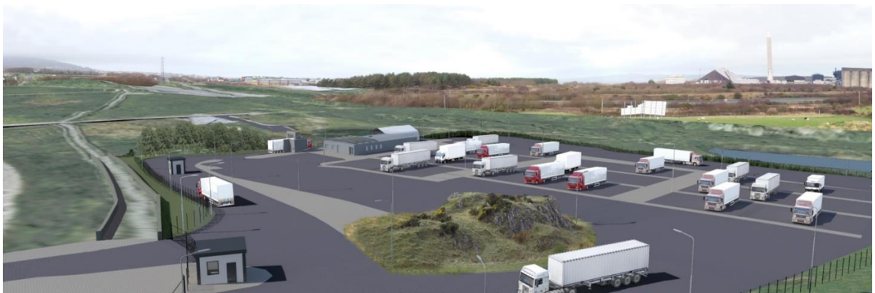
Figure 0-9 Aerial impression of the Logistics Centre
