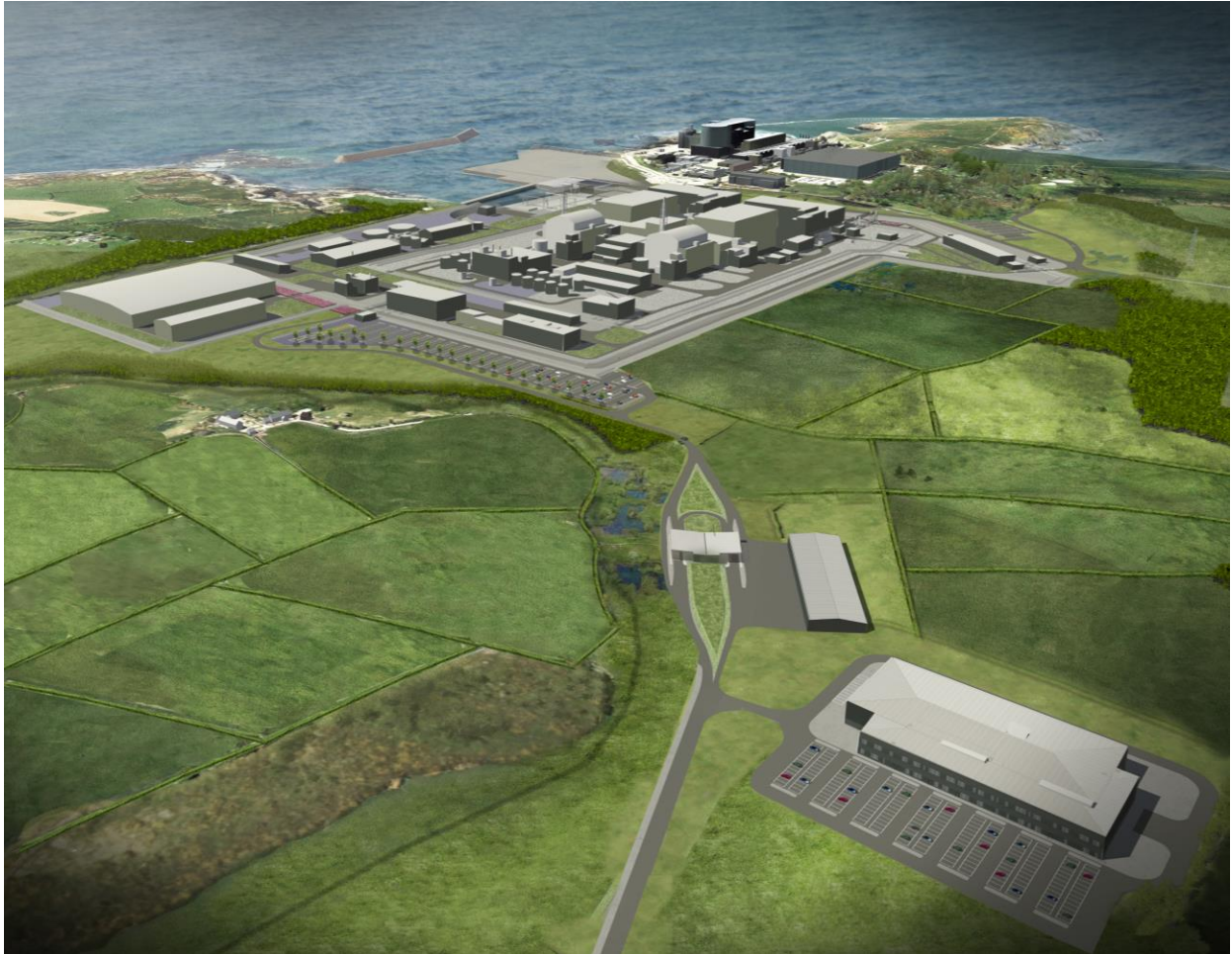
Figure 0-4 Aerial impression of the Power Station
